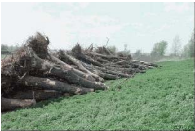
A stockpile of rootwads ready for installation
