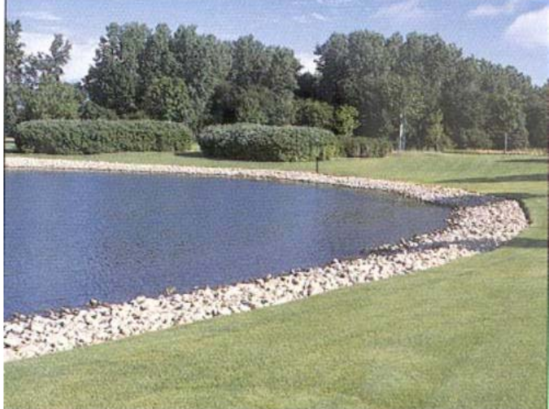
Riprap stabilizing a lake shoreline
