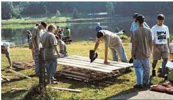
Building Fish Spawning Structures
