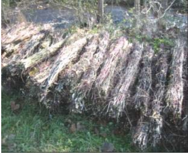
Live fascine bundles awaiting installation Source: F. X. Browne, Inc.
