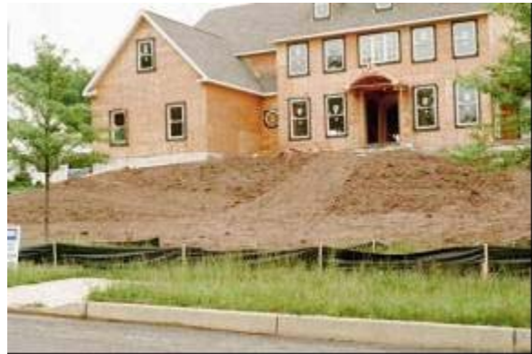
Well maintained silt fence Source: Edward Molesky, Aqua-Link, Inc.
