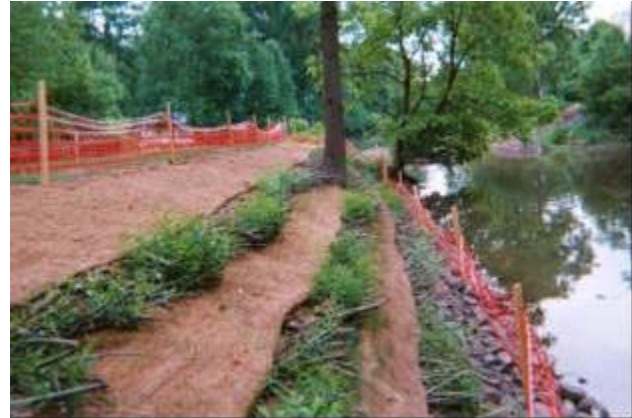
First year growth on willow and dogwood cuttings used in a vegetated geogrid installation on the East Branch Perkiomen Creek, Bucks County, PA Source: F. X. Browne, Inc.
