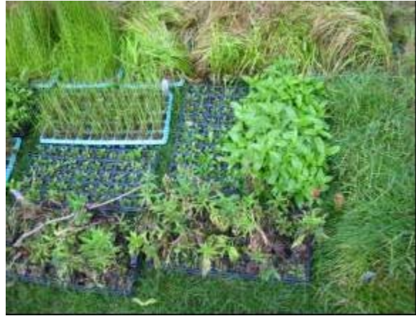
Native grass and wildflower 2 in. plugs awaiting installation. Plugs are a good way to establish native plants on a graded streambank.
