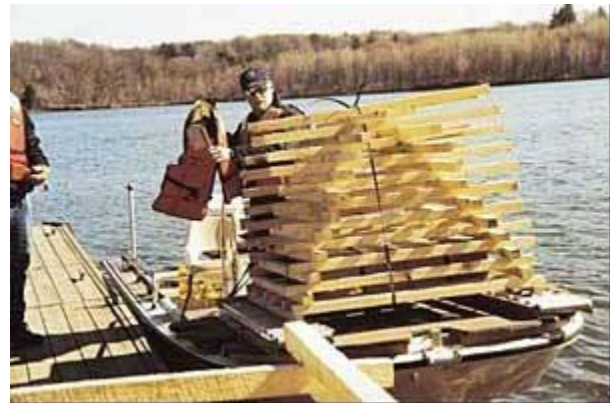
Porcupine crib habitat structure installation Source: PA Fish and Boat Commission
