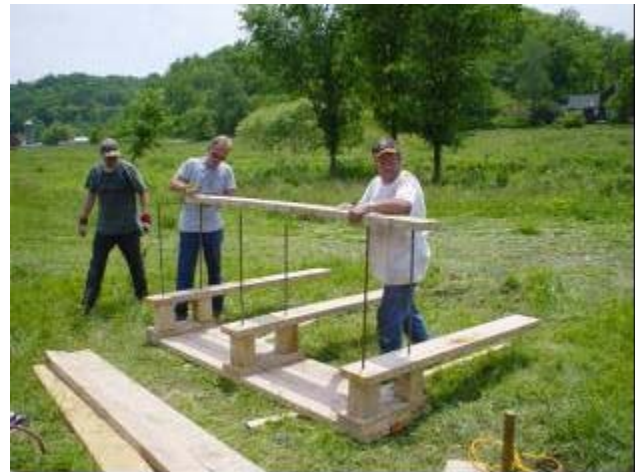
Construction of a LUNKER structure prior to in-stream placement.
