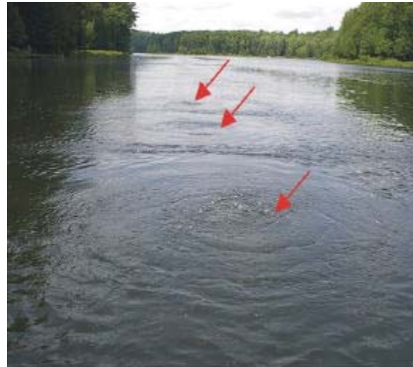
Plumes of air bubbles along an installed in-lake aeration line. Source: Ed Molesky of Aqua-Link, Inc.
