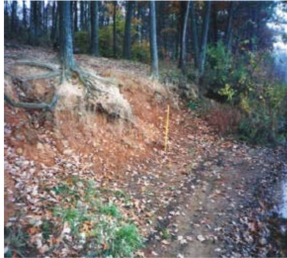
Severe lake shoreline erosion at Pinchot Lake in York County. Erosion due to wave action and heavy pedestrian foot traffic. Source: Edward Molesky of Aqua-Link, Inc.
