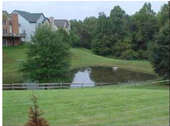
A wet pond in Fairfax County, VA Source: Fairfax County DPWES
