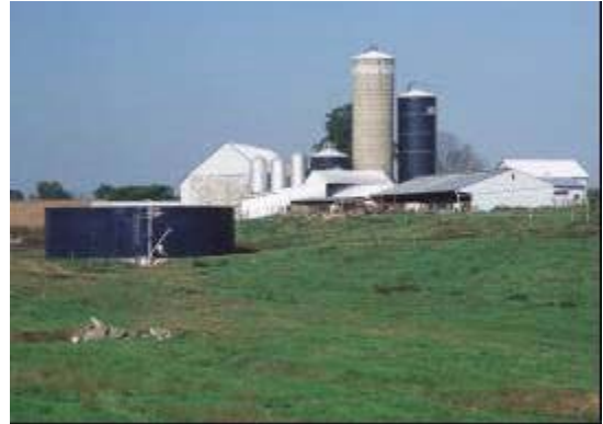
Manure Storage Tank Source: USDA NRCS
