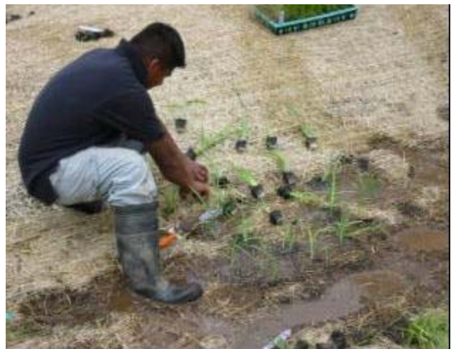
Installation of native herbaceous plugs through an erosion blanket
