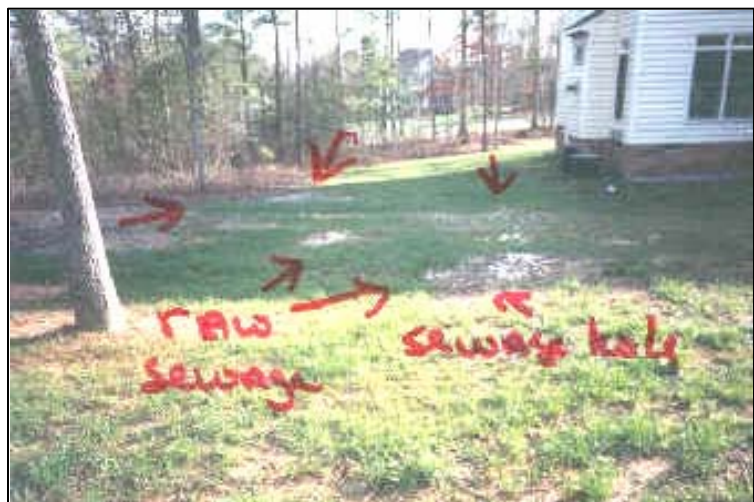
Failing Septic System Source: Anish Jantrania, Ph.D., P.E.
