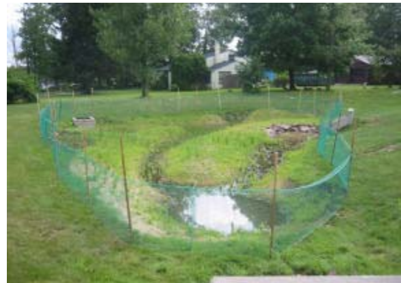
Constructed stormwater wetland treat parking lot runoff at F. X. Browne, Inc., main office in Lansdale, PA Source: F. X. Browne, Inc.
