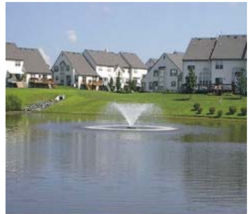
Fountain aerator installed in a stormwater retention pond in Bucks County. Source: Edward Molesky of Aqua-Link, Inc.
