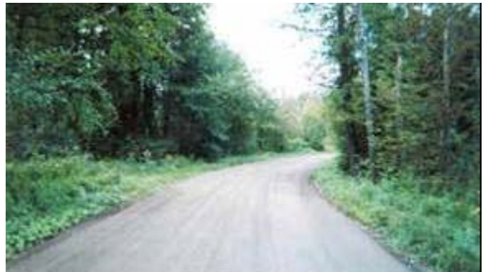
Properly constructed and maintained dirt road with well-vegetated road edges
