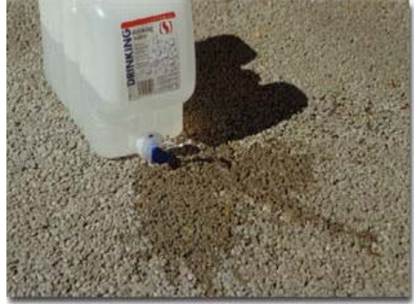
Porous concrete allows stormwater to rapidly infiltrate
