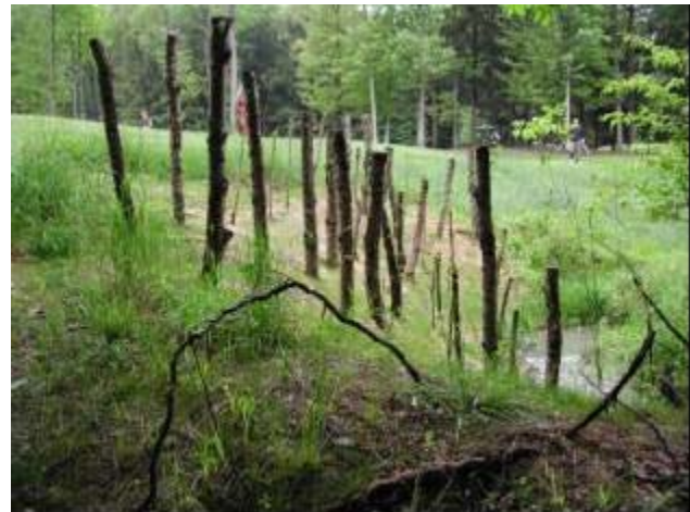
A completed dormant post stabilization system along Teedyuskung Creek, PA
