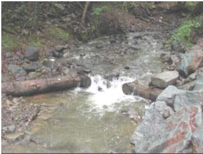
A double wing flow deflector on Teedyuskung Creek, Pike County, PA. Note the formation of a scour pool downstream of the structure.
