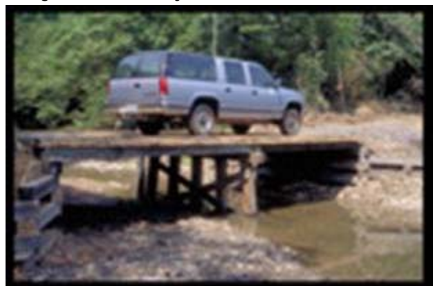
Bridge on a logging road Source: USDA Forest Service
