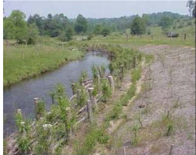
A completed dormant post planting along the South Branch Tunkhannock Creek five months after installation
