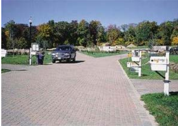
Pervious paving systems have open spaces between the paving stones to allow infiltration
