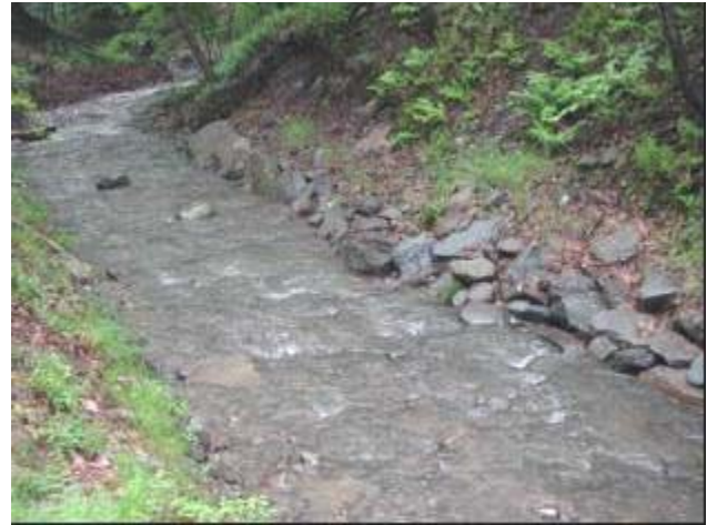
Completed boulder toe installation along Teedyuskung Creek, Pike County, PA.
