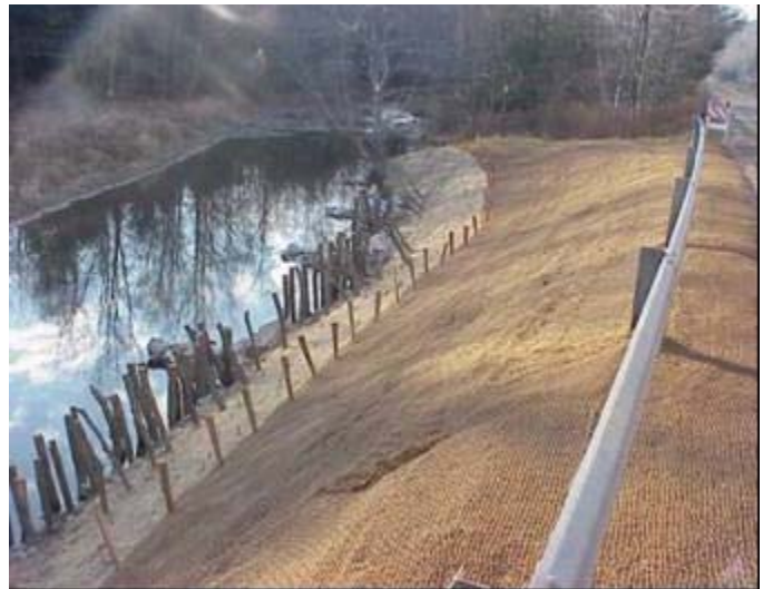
An integrated biostructural streambank stabilization project along the East Branch Wallenpaupack Creek, Pike County, PA Source: F. X. Browne. Inc.
