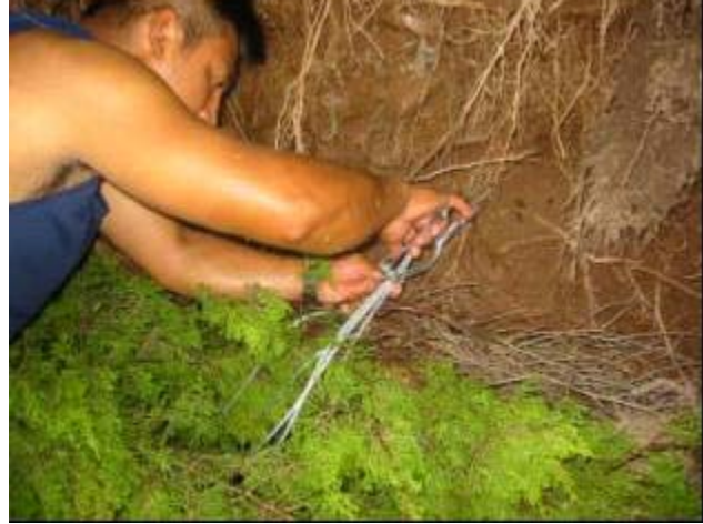
Cabling a tree revetment to an earth anchoring system
