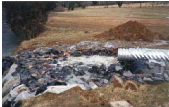
Hydraulic dredging: return water effluent following sediment removal in a sediment disposal basin
